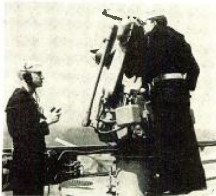
Gun control "talker" (l.) maintains contact with gun crew while operator tracks target
