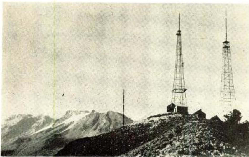
18,800 ft. Mt. Popocatepetl, once active Mexican volcano, is now the site of the highest TV transmitter in the Western Hemisphere. Located some 3,000 ft. below the volcano's summit at Paso de Cortez, about 50 miles from Mexico City, the 45 kw station is the most powerful in Mexico. Equipment development was by Federal Telecommunication Labs, Nutley, N.J., research division of IT&T.
