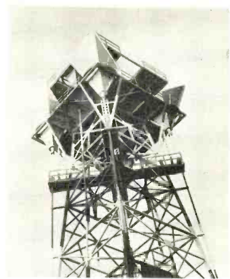
AT&T "horn reflector" microwave antenna installation is capable of handling 15,000 phone conversations and 10 TV programs at same time
