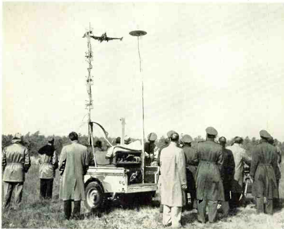
Field mobility of new control system for pilotless jet fighter-bombers is shown during U.S.A.F. acceptance trials. Guidance antennas are vehicle mounted; control box at right
