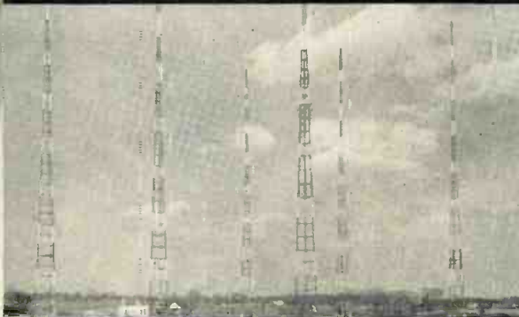
WFMJ-FM Truscon Self-Supporting Directional Towers, 400 Feet Tall
