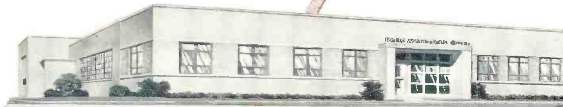
RMC Plant and General Office at Chicago, Illinois
