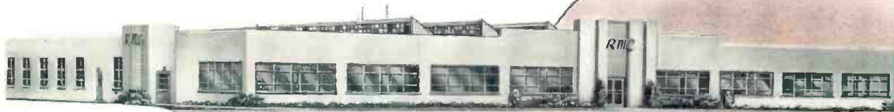
RMC Plant at Attica, Indiana
