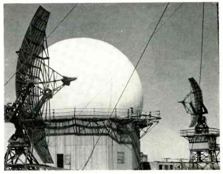
Three versions of new radar height finder made for U.S. Air Force are (I) mobile unit, (c) radome for radar in Arctic climates, and (r) unit for fixed installations in temperate regions
