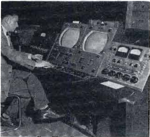
Control desk for "package" TV station allows one operator to handle film and net programs
