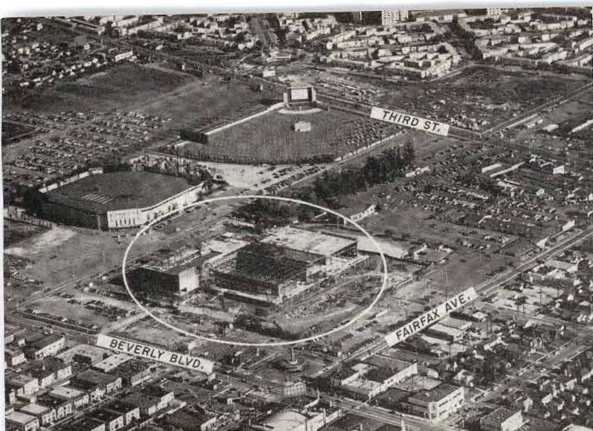
Fig. 1: CBS TV City in Hollywood, Cal., photographed during an intermediate stage of construction
