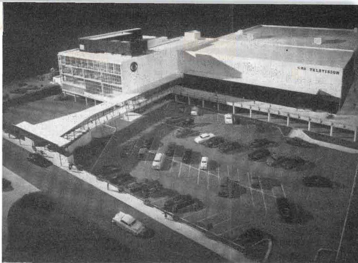
Fig. 2: Model shows offices (l) and wing (r) containing two audience and two non-audience studios
