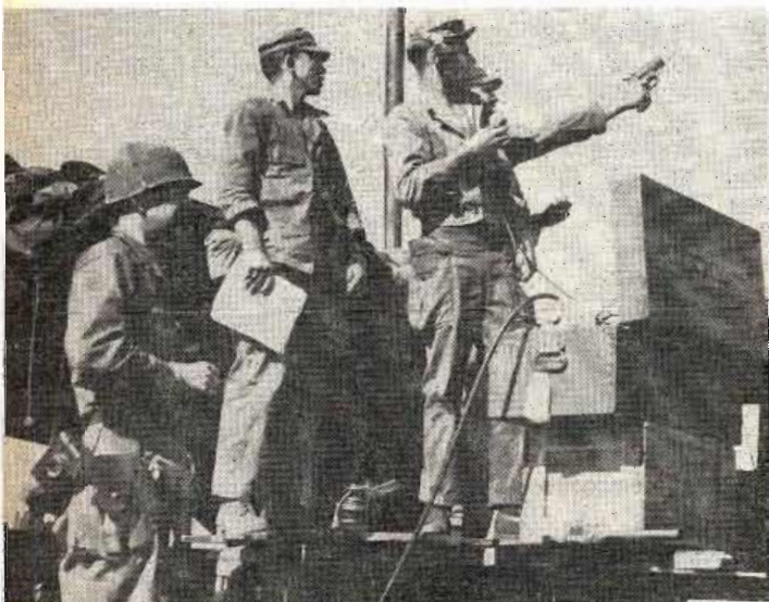
Makeshift control tower being operated by Airways and Air Communication Service (MATS) personnel at Kimpo airfield in Korea. Signalling equipment includes a Very pistol for signal flares, heliograph for visual signals and a type AN/CRC-2 radio set for direct communication with planes.
