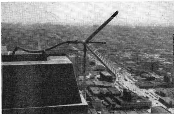
← Fig. 3: (left) Transmitting antenna mounted on Power and Light Building. Note size.
