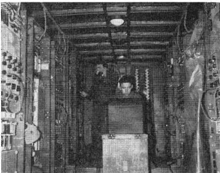
Signal Corps men at work in the carrier van at U. S. Eighth Army Headquarters, Taegu, Korea. Placement of heavier rack mounting equipment in motor trucks minimizes time required for installation and dismantling when Headquarters relocates.
