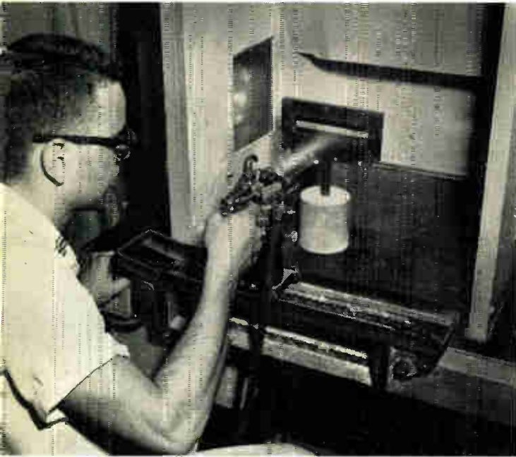
First step: Spraying the cathodes with a coat of barium-strontium-calcium-carbonate.
