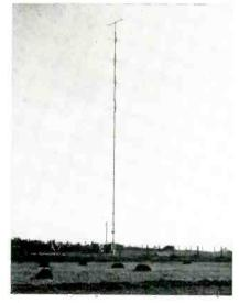
The BBC is using "translator" stations to relay television programs to outlaying towns in England. Pictured below is the receiving and transmitting aerial mast on Creteway Down. The television translator units can be seen near the base of the mast.
