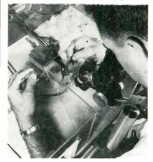
At Bell Telephone Labs T.B. Light is using a newly developed method of compression bonding to join gold leads to a transistor.
