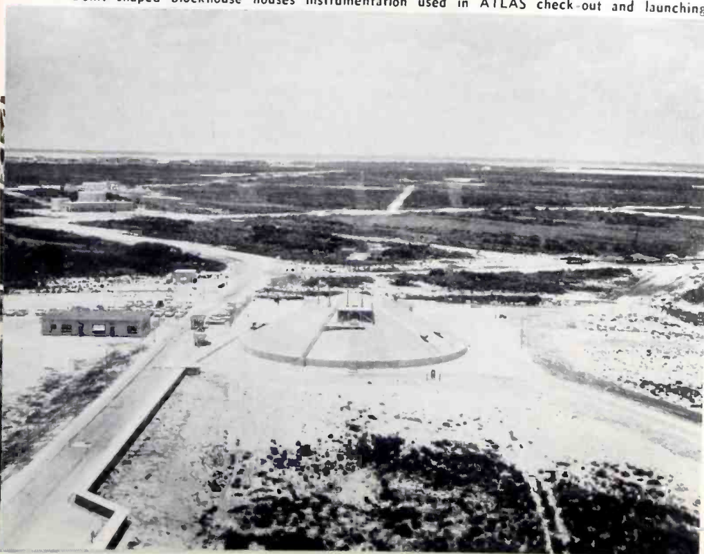
Dome-shaped blockhouse houses instrumentation used in ATLAS check-out and launching.
