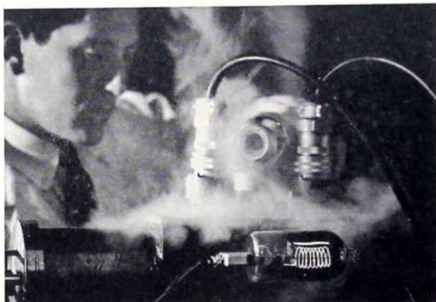
Advanced research on the Maser (Microwave Amplification by Stimulated Emission of Radiation) performed by the R&D Laboratories is directed towards applications of a portable, airborne Maser for missiles and aircraft.
