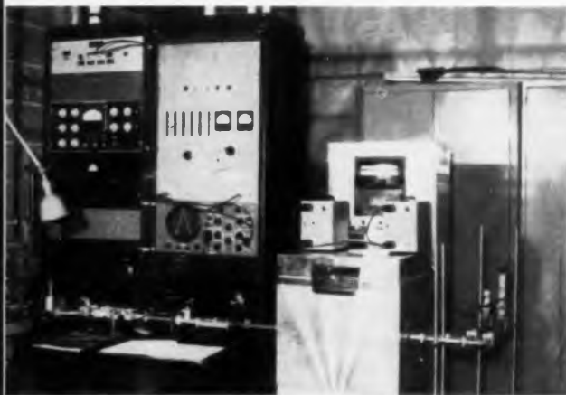
Fig. 1: Equipment and plumbing used in high accuracy cavity test.
