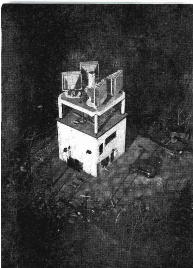
(Left) Typical Bell System microwave relay station used for TV transmission over some 360 route miles. (Right) Cut away view shows location of emergency power equipment and storage batteries on first floor, radio equipment on second, and directional antennas on second roof
