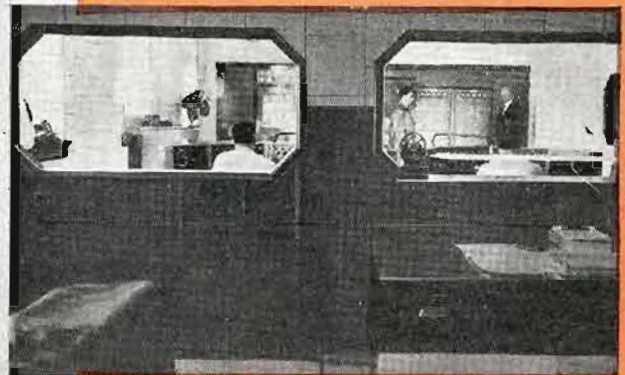
RADIO ROOM is soundproof and air conditioned for top efficiency. In foreground are Remote Control Consoles for direction of police and fire department mobile units. Standing by Federal transmitters are R. E. Altoonian, Federal Engineer, (left) and Captain William E. Taylor, head of Baltimore's Communications Division.
