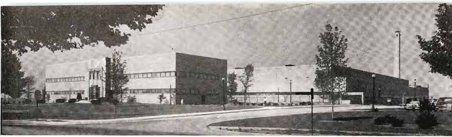
Western Electric's new Allentown plant, designed and built by the Austin Co., houses upwards of 2500 workers who can perform the hundreds of processing and assembly functions involved in the design and production of vacuum tubes and other communications equipment
