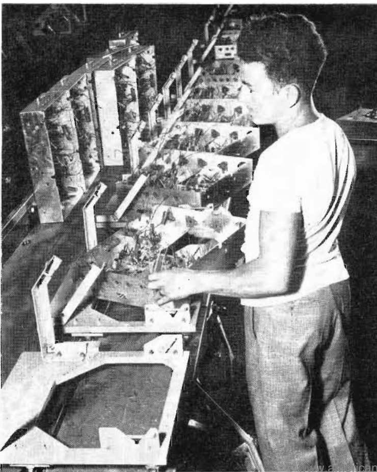
BELOW: Start of assembly line. The chassis with some parts already riveted in place are loaded on special aluminum cradles on casters which run in metal tracks. Chassis operations follow
