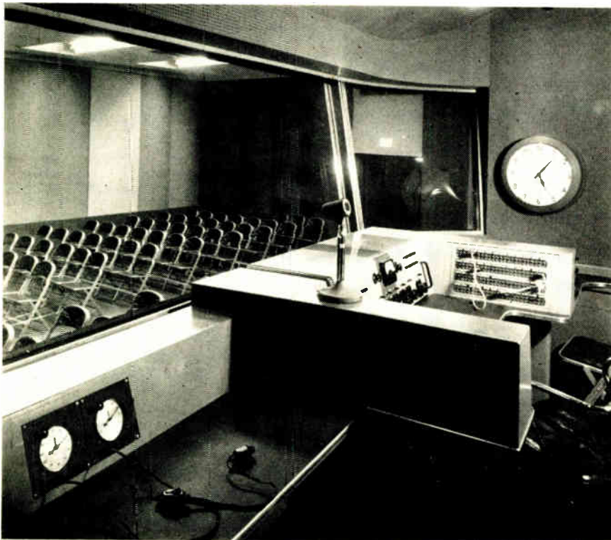
Typical studio control booth. Note novel stop-watch with inverse numbering to save production engineers a mental operation in figuring "seconds to go"
