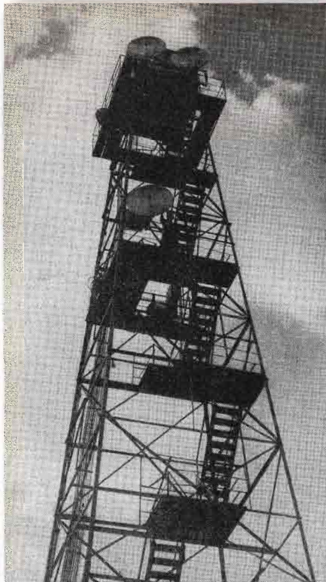
Repeater station tower at Ten-Mile Run
