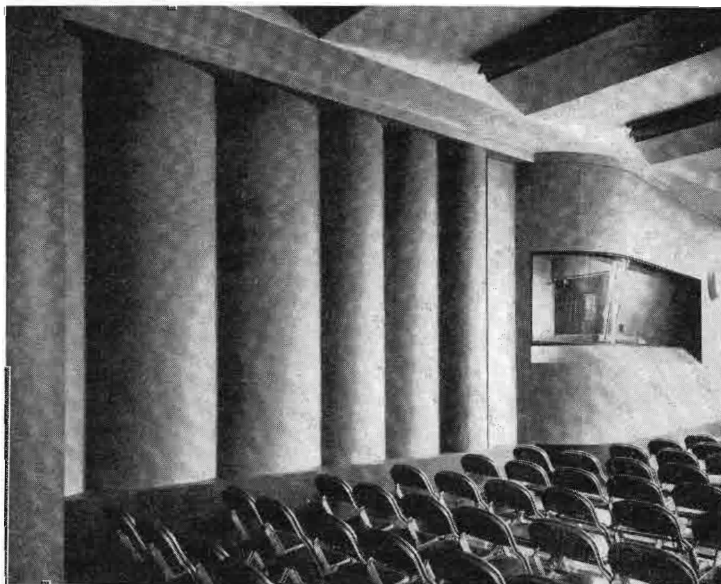
Polycylindrical side-walls and splayed ceilings keynote the studio design at WNEW
