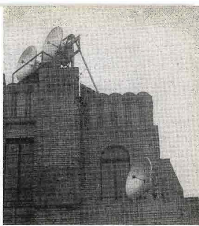
Television signal distribution amplifier antenna installation at Philadelphia end
