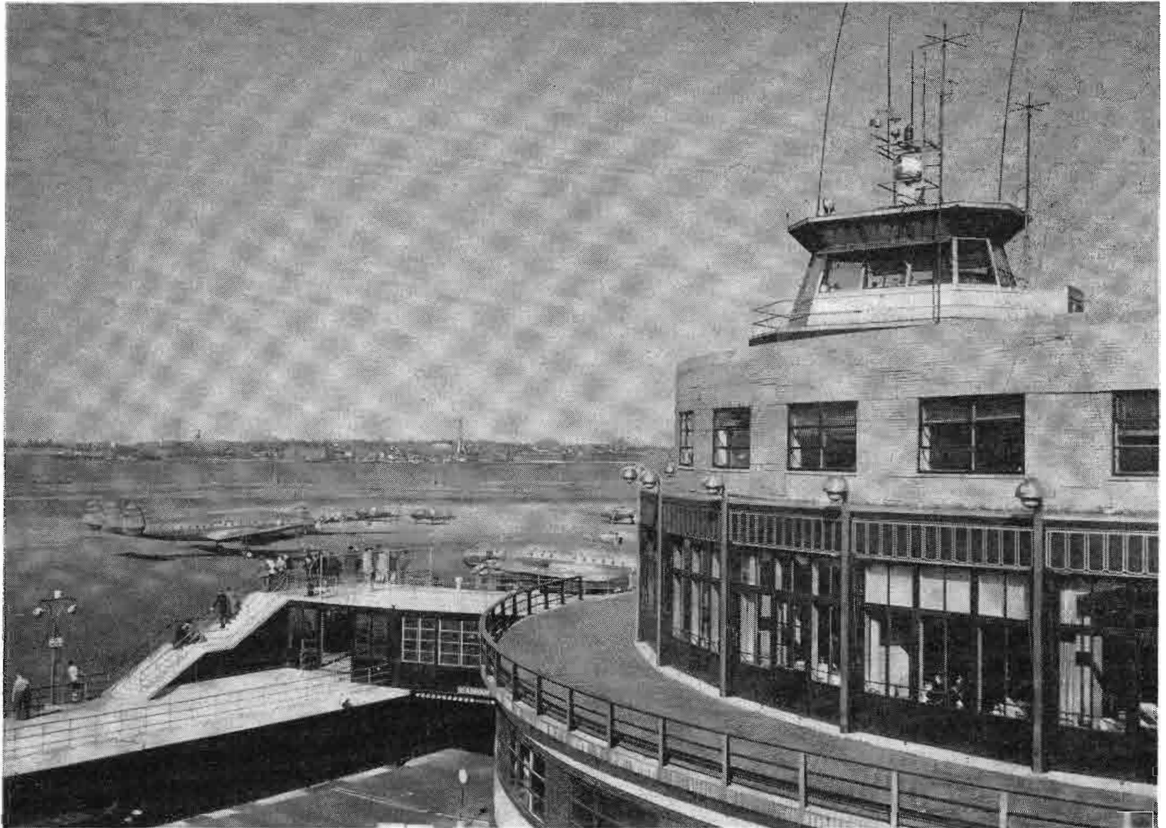
LaGuardia field administration building and control tower in New York. The inclination of tower sides and roof give widest vision
