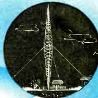
1930 Half-wave vertical radiator, now in general use, was developed into practical form. It greatly improved signal output of broadcast stations.
