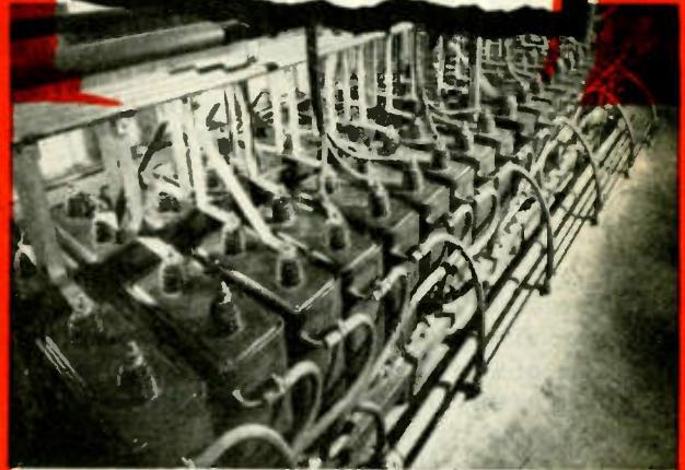
"Made induction heating practical"—This bank of G-E water-cooled capacitors is used with two Ajax-Northrup induction-type steel furnaces in a Western metals plant.
