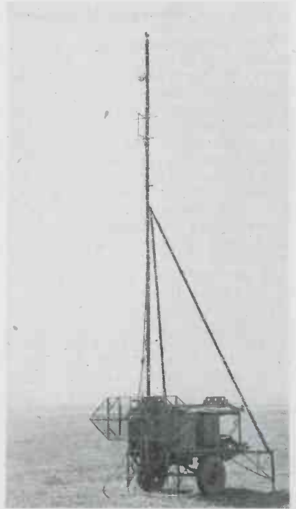
Development model of glide path transmitter
