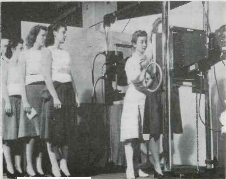
Method of mounting phototube camera on any standard fluorographic hood. Right—Timer in position on camera as subjects are positioned for making chest X-rays on 16mm. film
