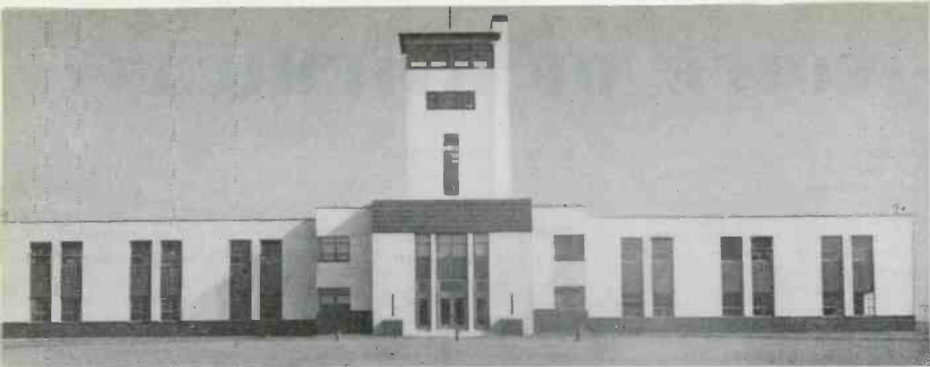
The building that houses the Bethany installation is two separate units, an administrative section and a transmitter section, the former having a four story tower that serves as a guard station and for a beacon, quarters for resident engineers. The transmitter section is 175 x 75 ft.
