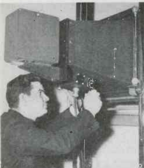
Method of mounting phototube camera on any standard fluorographic hood. Right—Timer in position on camera as subjects are positioned for making chest X-rays on 16mm. film
