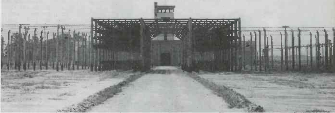
The main antenna switching station provides facilities for connecting the transmitters to the 27 radiators that are used, all being of the rhombic type. All are four wavelengths long. To change frequency two men are needed, one at the transmitters and the other to connect proper antennas
