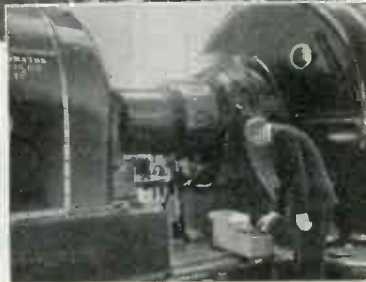
Measuring insulation resistance on generator.
