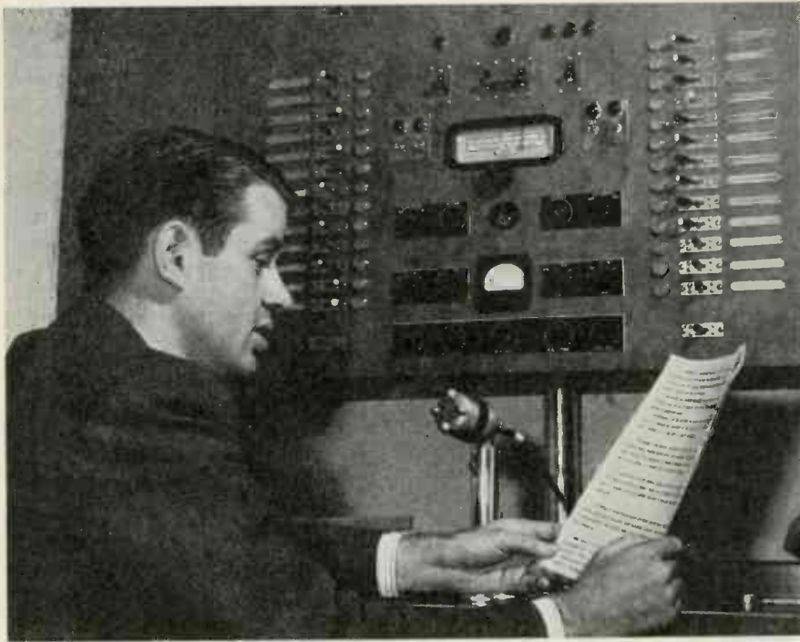
CONTROL PANEL for the PA system in the factory buildings of North American Aviation
