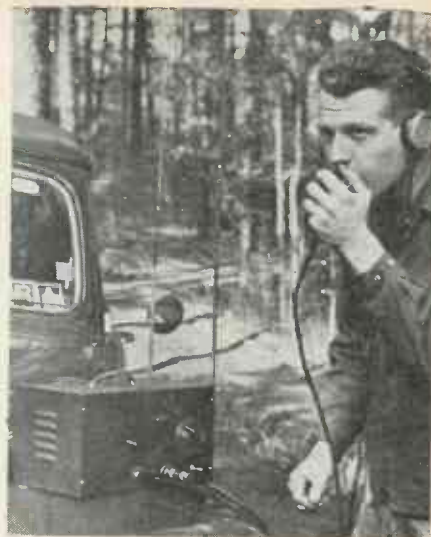
MOBILE WERS stations report direct to local control center
