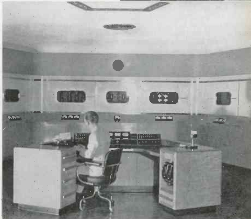
Base insulator for tower, transformer for tower lights and searchlight. Below—Control room for WABC transmitters—the 50 kw main unit and the 5 kw standby outfit for emergency operation
