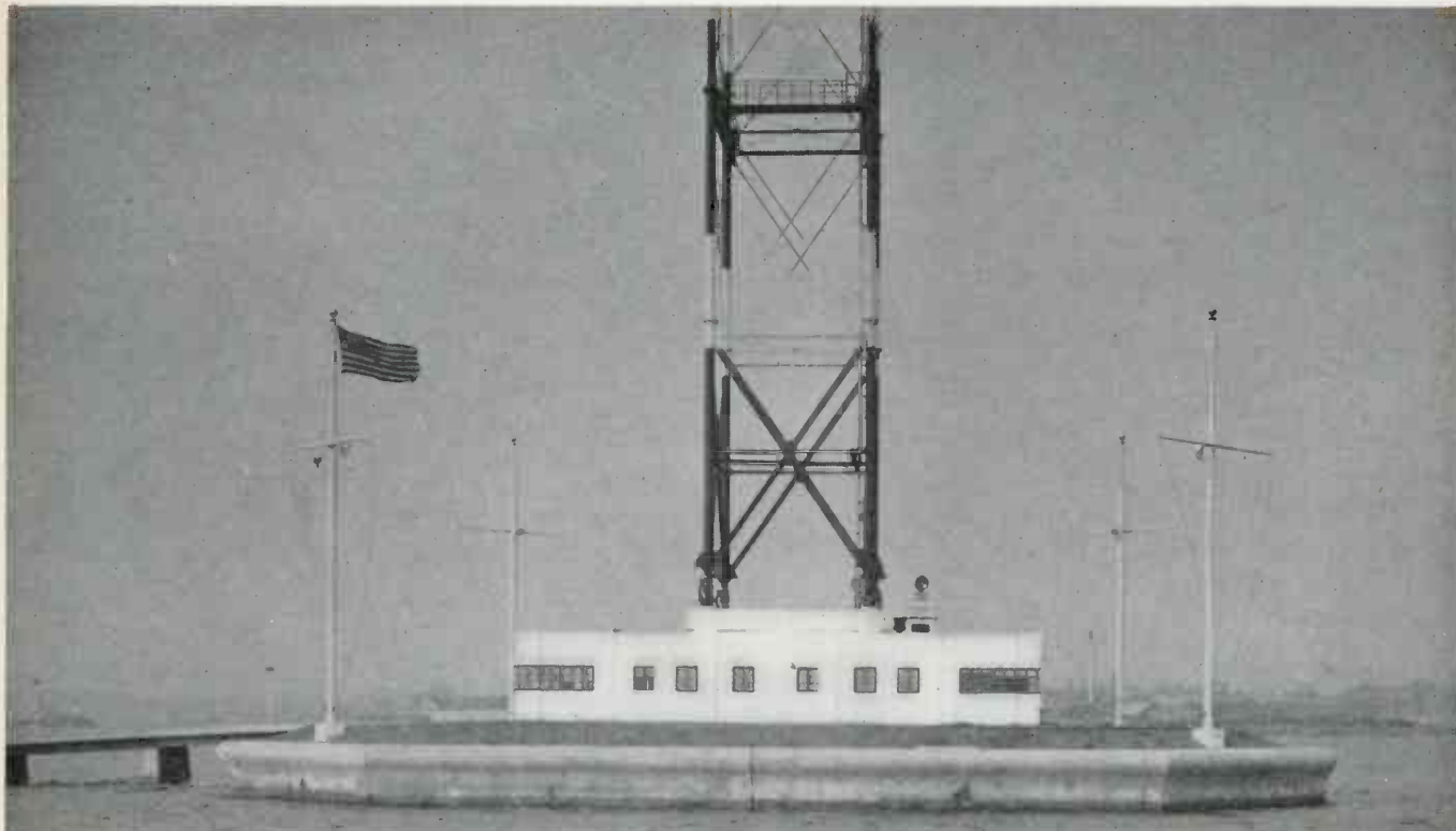
Close-up of Columbia Island in Long Island Sound, showing reinforced-concrete bulkhead designed to break up wave action
