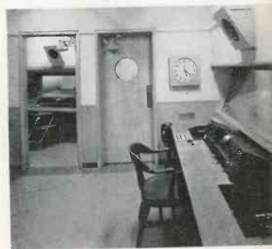
▼ Below—Close-up view of control desk. Monitor speaker is mounted above. Note the convenient layout and broad view of the studio
