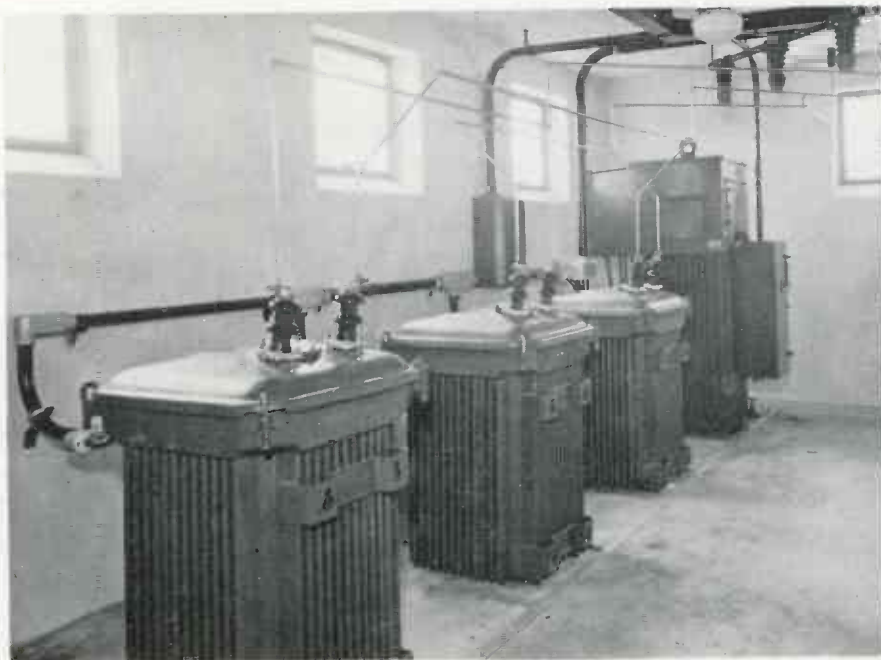
↑ The high-voltage transformers for plate supply of final amplifier in the basement of the transmitter house
