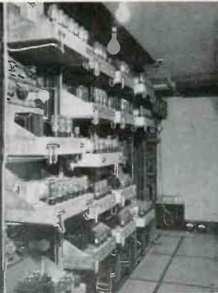
The racks of vacuum-enclosed forks and associated amplifying tubes
