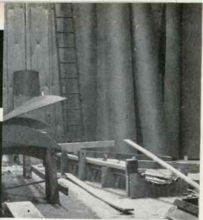
Construction of convex panels. Plywood sheet on the left is just in process of being bent
