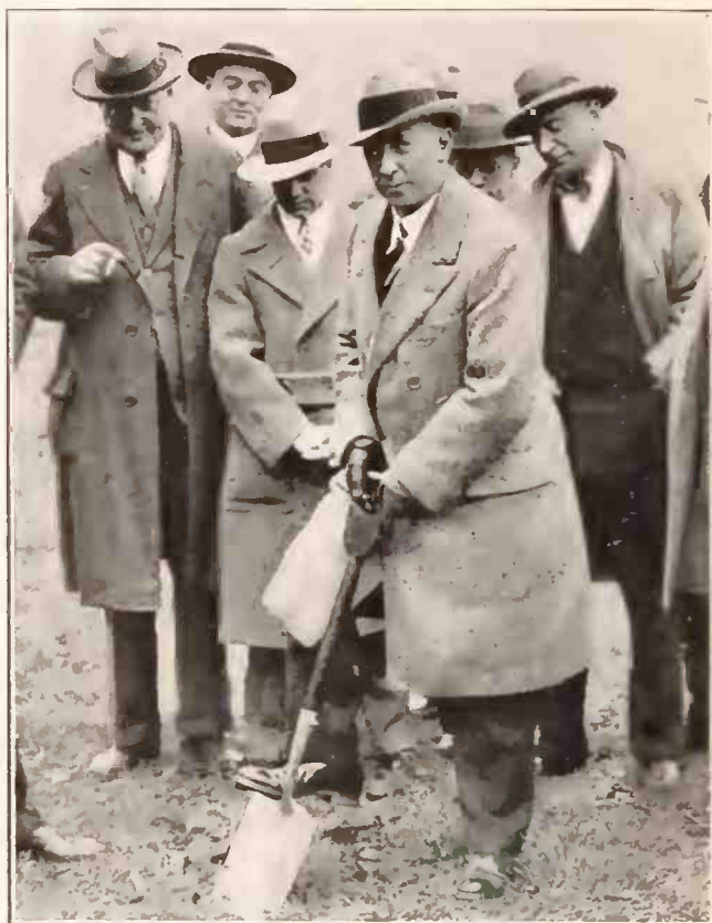
Above—A. Atwater Kent using a silver spade to turn over the first spadeful of earth for new $3,000,000 factory
