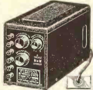
VESTA "B" UNIT Socket Power with Automatic Relay.
