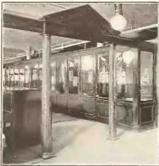
Note the Battery of Booths
