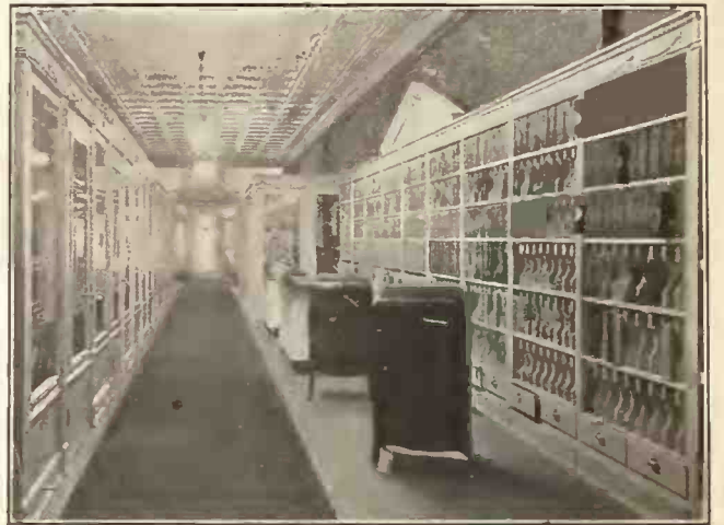
Booth Installation for Deep Store
