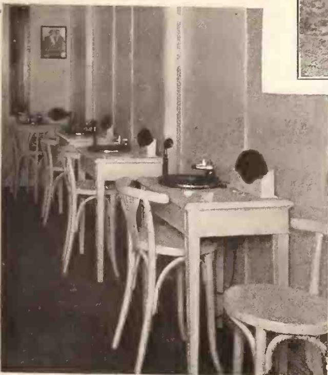
A CORNER IN STORE SHOWING SEVERAL X-T AUDAK UNITS
