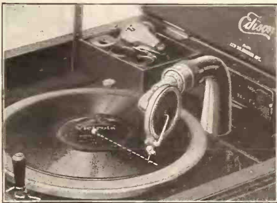
SHOWING POSITION FOR PLAYING VICTOR AND OTHER LATERAL CUT RECORDS
