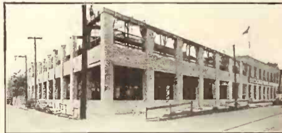
New Buescher Building Being Constructed
