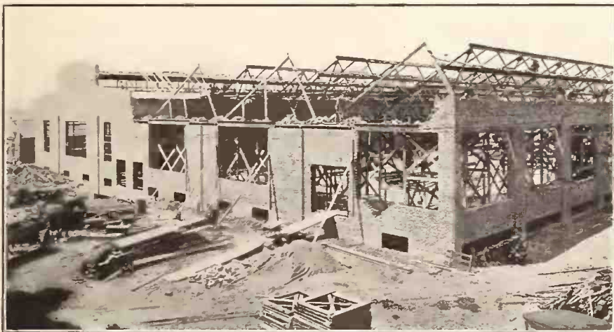
Photograph of Addition to Brunswick Record Plant Taken Some Time Ago
