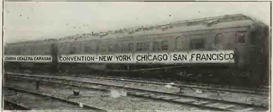
The Edison Caravan Train Under Way
