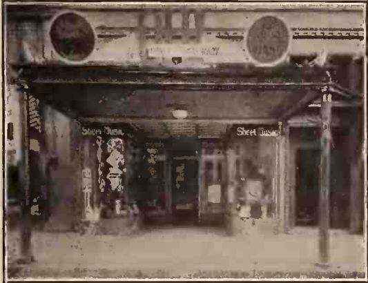
Exterior View of Dreibelbis Song Shop
