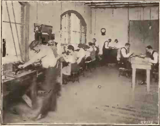
Corner of the "Don" Factory
