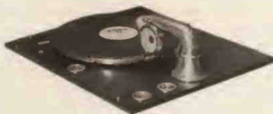
Showing the Empire Reproducer turned back to permit insertion of needle
