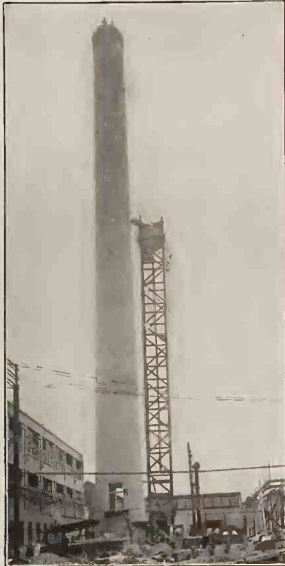
Chimney for New Edison Power House
