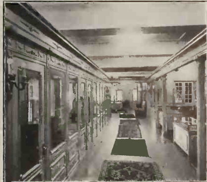
Looking From Rear to Front of Salon
