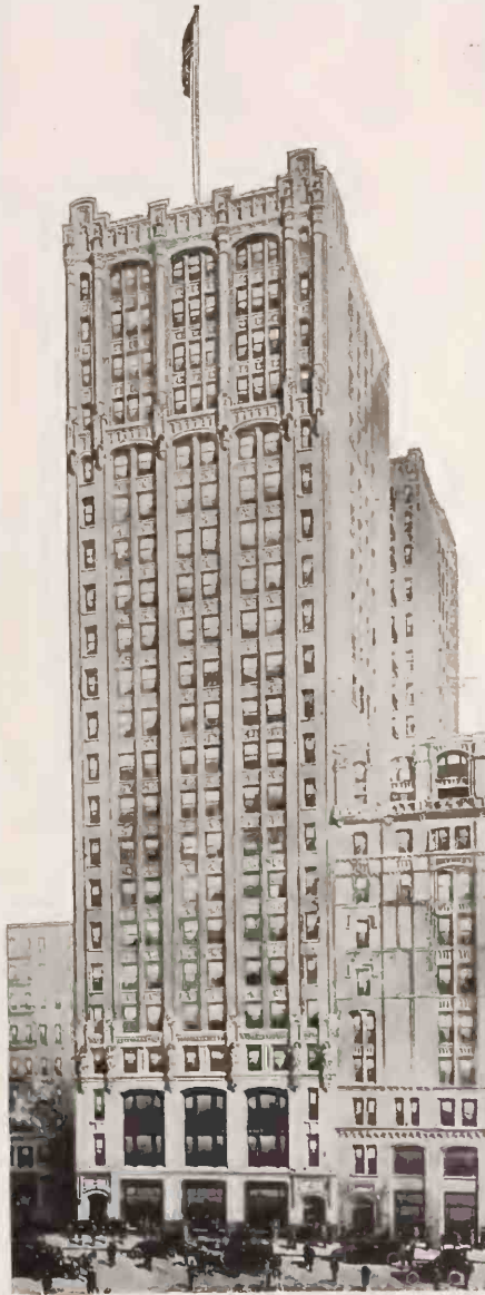
New York Talking Machine Co.'s New Home. work and concentration in reorganization. The up-to-date way to guard against this is the installation of one's business in a building as thoroughly fire-proof as human ingenuity and money can make it.
