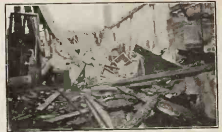
View of Display Rooms on Fourth Floor.
