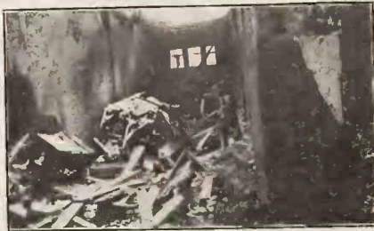
McGreal Office in Burned Building.
