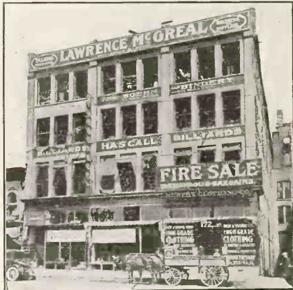
The McGreal Building After the Fire.
