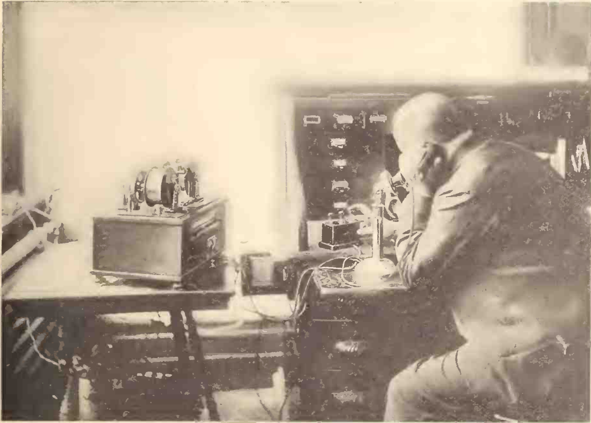
Telegraphone making a record of conversation over the telephone in a Wall Street office. Everything that passes over the line is stored on the spool wire of the machine for permanent record.
