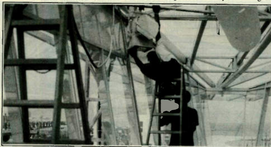
NBC Morning Show set. Tilting the glass out drew the ire of many old-school lighting directors.
