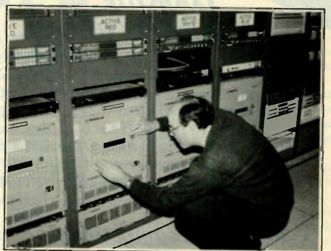
John Bracco checks out one of NBC's four Thomson standards converters at the IBC facility in Barcelona.
