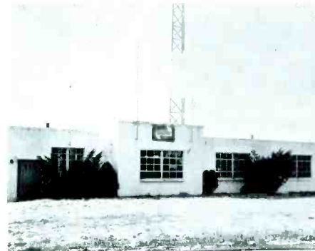
OPERATIONS of Mobile Radio Dispatch Service, Inc., are coordinated in this building located in East Brunswick, N.J.
