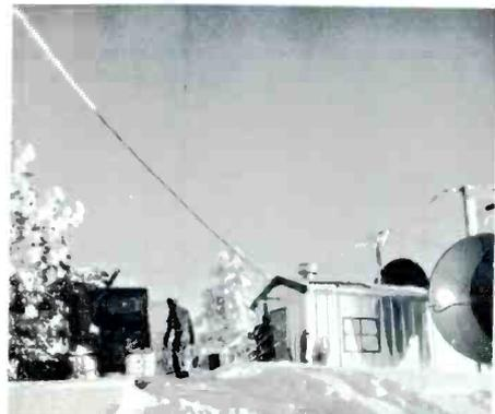
Power lines coated with ice to the thickness of a man's arm, snow four feet deep on the level at Monida Pass location near Montana-Idaho border. Snow weasels bring in men and supplies. Note 10 foot dishes, painted black, to resist frosting conditions.
