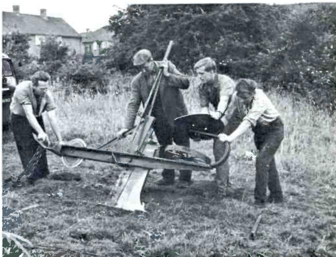
Getting set for a mole-ploughing exercise. This picture clearly shows the cable laying mole-plough, and the operation is under the direction of George Henry (Relay) Limited, Relay Contractors, of Eynsham, Oxford.
