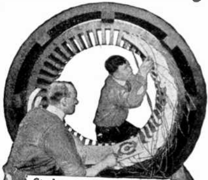
Student winding a Stator in The Great School of COYNE
