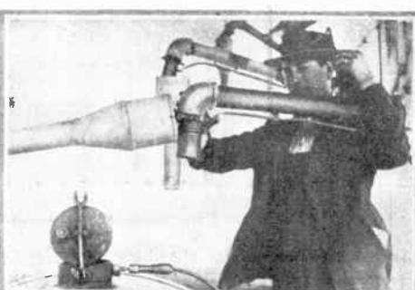
The operator is preparing to fill the tank which has been protected by the insertion of the anti-static plug. It will be noted the cap is wide open.
