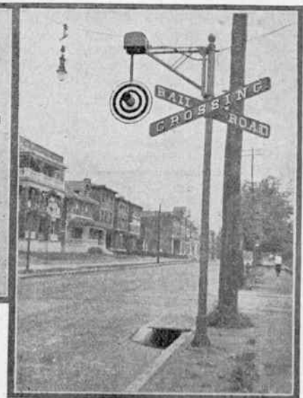
The electric flagman. This semaphore moves back and forth when a train is approaching, so as to give an unmistakable indication of the approach of a train on a crossroad.
