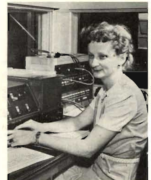
During World War II, ladies replaced many of the men who entered the armed services. This is Margaret Lowe who manned the control panels during the war.
