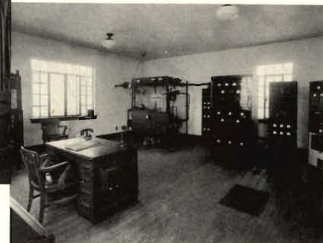
As Radio listening grew in popularity, WWVA began to improve its facilities and the transmitter site was moved to a hilltop near West Liberty, West Virginia. This view shows WWVA's 5,000 watt transmitter at that site.
