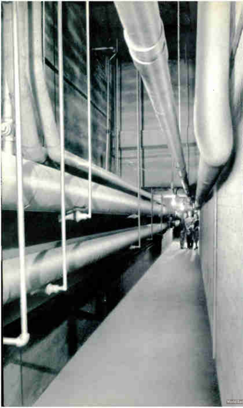
This underground service tunnel carries heat, hot water and refrigeration to the Radio City building.
