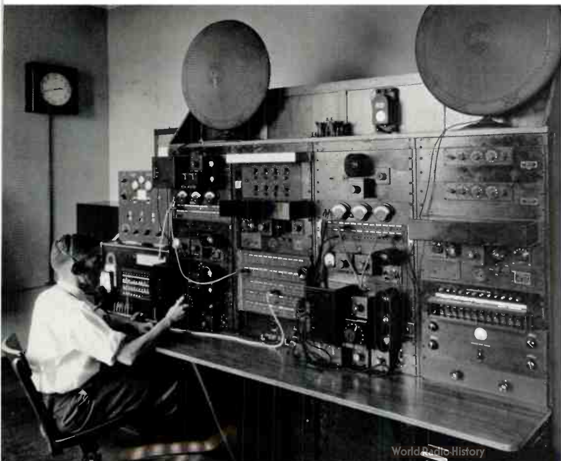
▼ The master control room adjacent to WTIC's sixth floor Grove Street studios. By 1929, the first RCA 50,000-watt transmitter (known as "Old Number One") was on-line at WTIC. Programs coming in from the studios were amplified and sent by telephone lines to the Talcott Mountain transmitter 12 miles away. That's Bob Coe, Engineer, at the controls.
