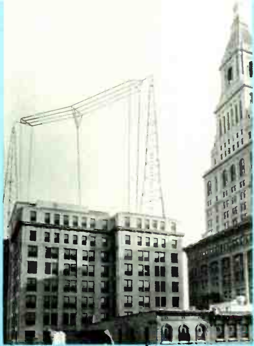
▲ A view of Hartford circa 1925. To the right, The Travelers Tower. To the left, the Grove Street building with WTIC's twin towers and T-shaped transmitting wires.
