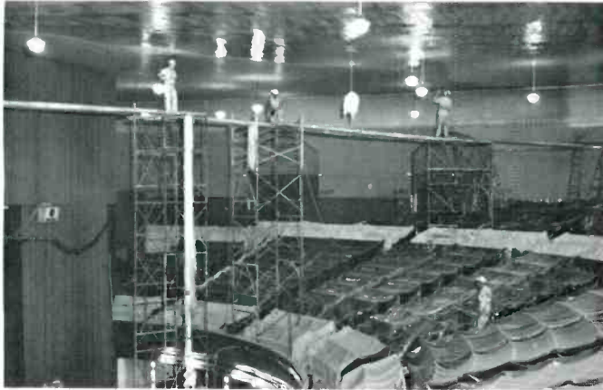
Even the ceiling gets dressed up. The Opry House ceiling, long dark in color, is given a gold paint job to brighten the surroundings.
