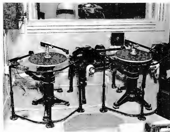
Engineering-wise these two strange-looking pieces of equipment are important in our history. They were the first turntables which played records at a speed of 33-1/3 rpm—a revolutionary development at that time.
