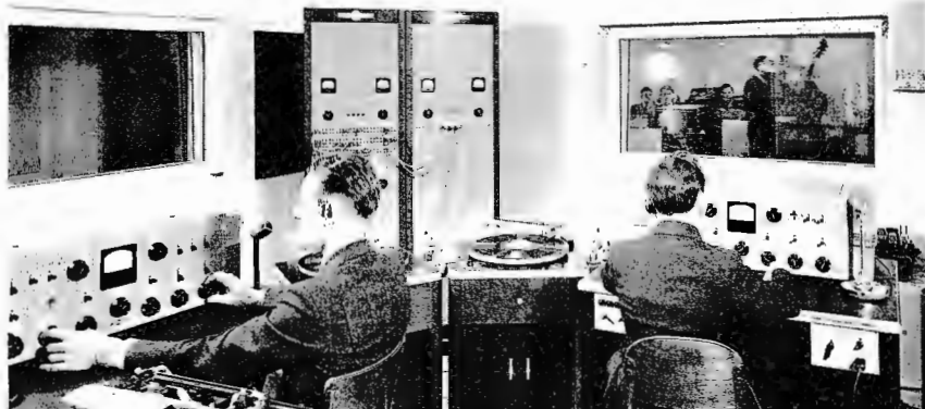
The Master Control Room is the nerve-center of any radio station, and by 1938, new equipment gave us this modern look. Ever-expanding live programming, on-the-spot broadcasts, news, music and network shows all were supervised here. This demanded an engineering staff of 12 men (large for those days). Shown here at the consoles are Dean Harger (now in his 26th WMT year), left, and Bob Besser, controlling an early broadcast by Ralph Slade's orchestra.
