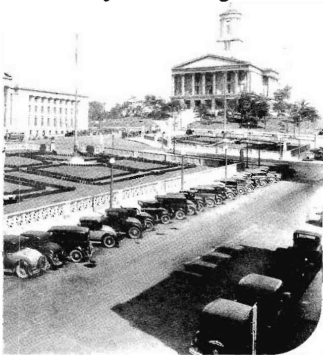
the State Capitol Building and War Building.
