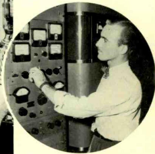
After servicing Sonar equipment in the Navy Harry Wingarter joined the staff of WKMH. He is shown here adjusting the phasing equipment which controls the station's four tower array.
